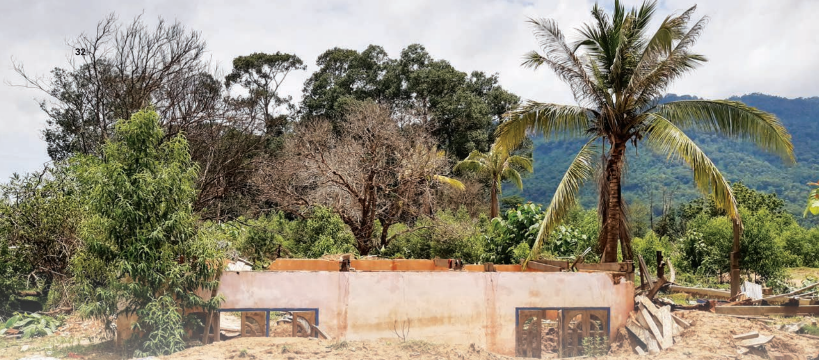
Damaged houses, Ban Tha Sangchan (Photo Credit TOE, June 2019)
