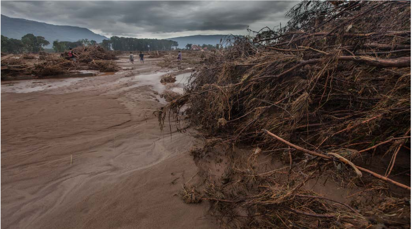
Impacts of the dam collapse in Ban Hinlat-Tha Sangchan. (Photo Credit Roengrit Kongmuang, July 2018)
